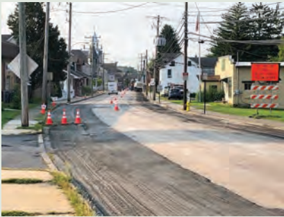
Milling and paving on Main St and Chestnut. Line painting on Main and ADA Ramps on Barrall St.
