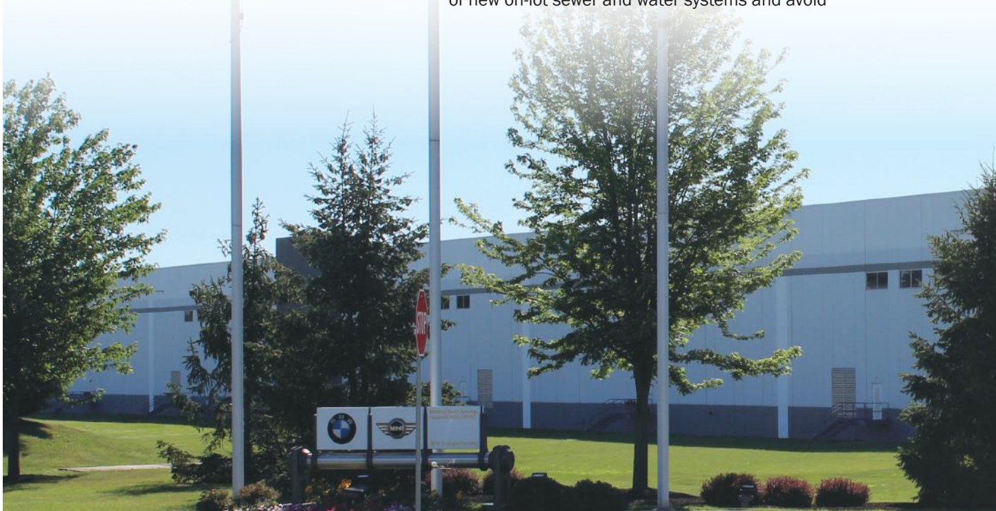
The BMW of North America warehouse in Lower Nazareth Township features some of the design elements, energy-efficient lighting and locally sourced materials recommended for warehouse development in the Nazareth Area.
