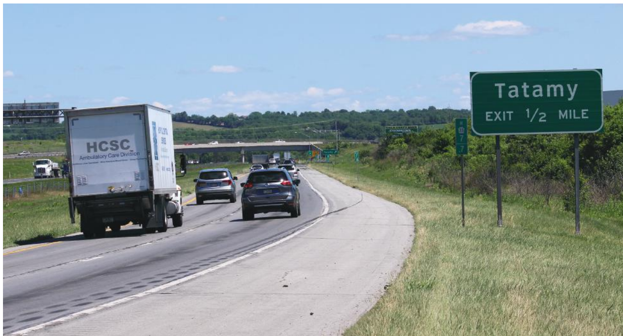
The Tatamy interchange was added on Route 33 to accommodate growing logistics development.
