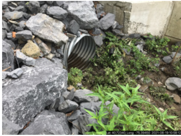
Photo #: OF-3 11 Outfall (Field)-003 Description: Outfall 003 Photo taken by SCOTT CONFER
